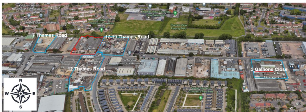
Figure 2: Google Earth screenshot showing the location of the neighbouring site with relevant planning history
